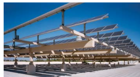
Stelling Parking Structure (top image); Stelling Parking Structure Rooftop Photovoltaic Panels (above)
