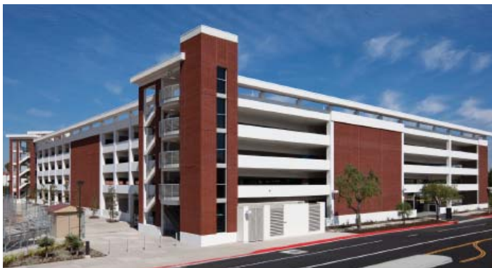
El Camino College Lot H Parking Structure (Photography by RMA Photography, 2009)
